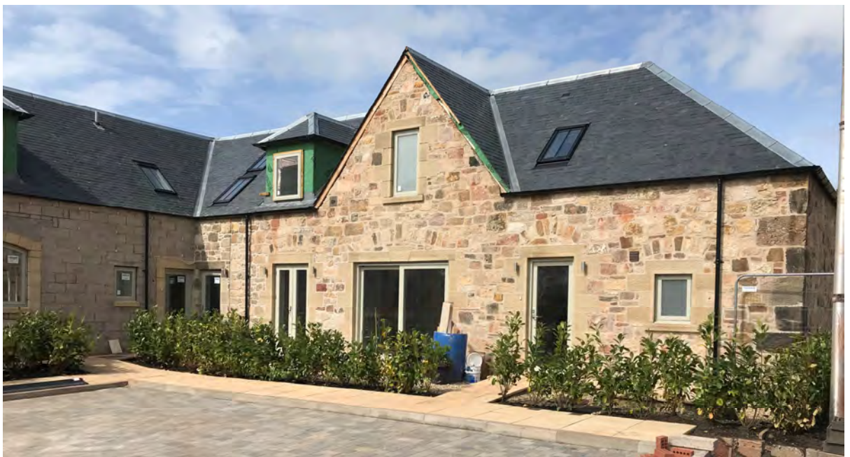
Figure (vi) View of Brunstane Steading Phase 3 Courtyard Looking South-west. (Currently under construction)
