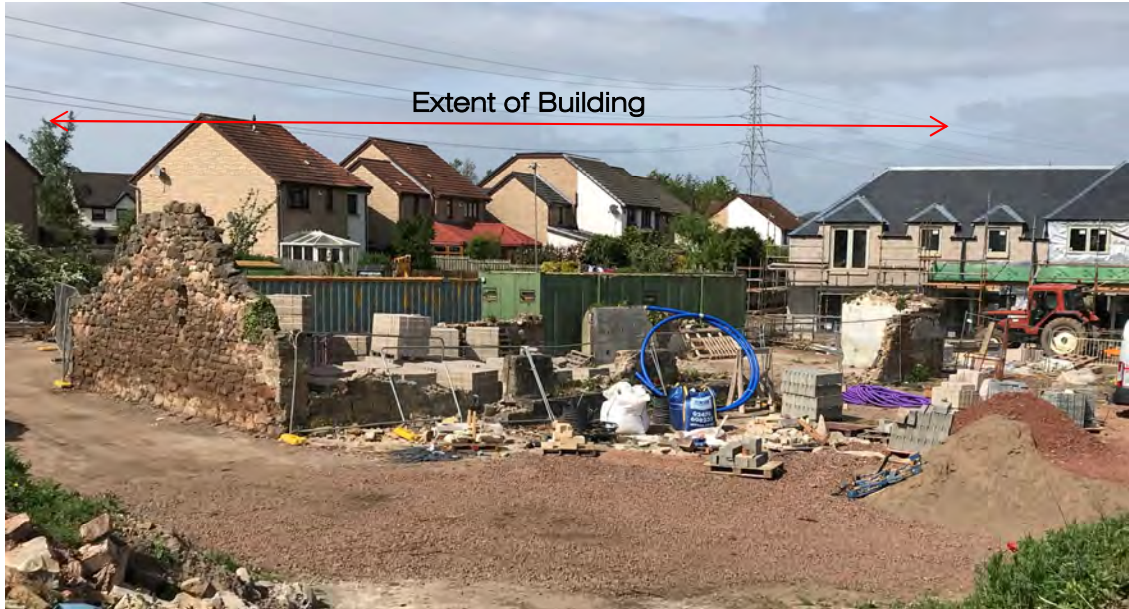
Figure (vii) Existing Building Looking South-west.
